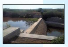
variety of materials, including clay, stone and cement. Earthen check dams, are cost effective and easy to construct. Masonry and reinforced cement concrete (RCC) structures, require some degree of construction experience and monetary inputs.
